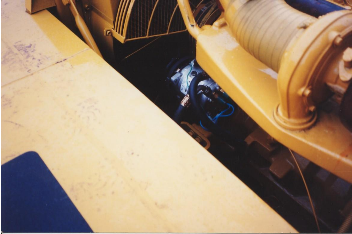
Compressor in place. View from underneath.
